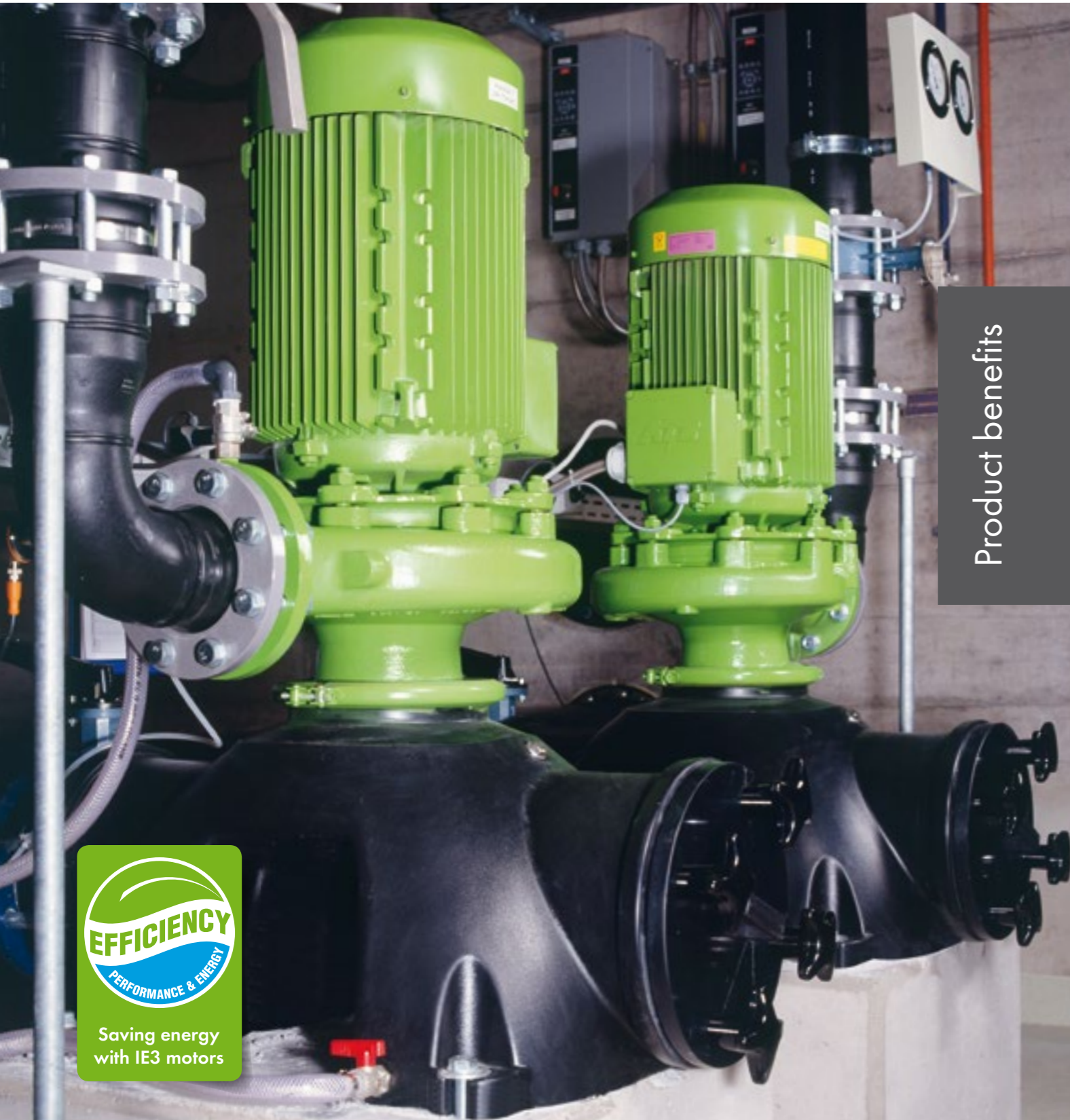
Fig.: Optimo-F pool water circulation pumps in a public swimming pool
